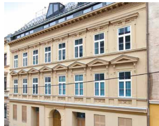
The facade of the former suburban property after its prize-winning renovation
