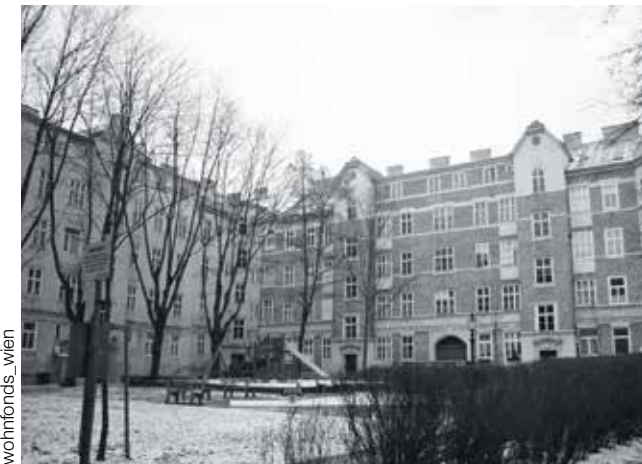
Lobmeyrhof in Ottakring: Interior courtyard before the renovation
