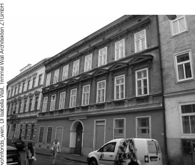
Facade of Dingelstedtgasse 12 before the renovation
